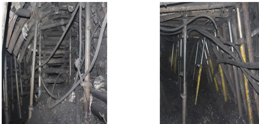
Fig. 1. Current support conditions at the coal face-roadway intersection and ahead of the coal face in some underground coal mines in Vietnam
