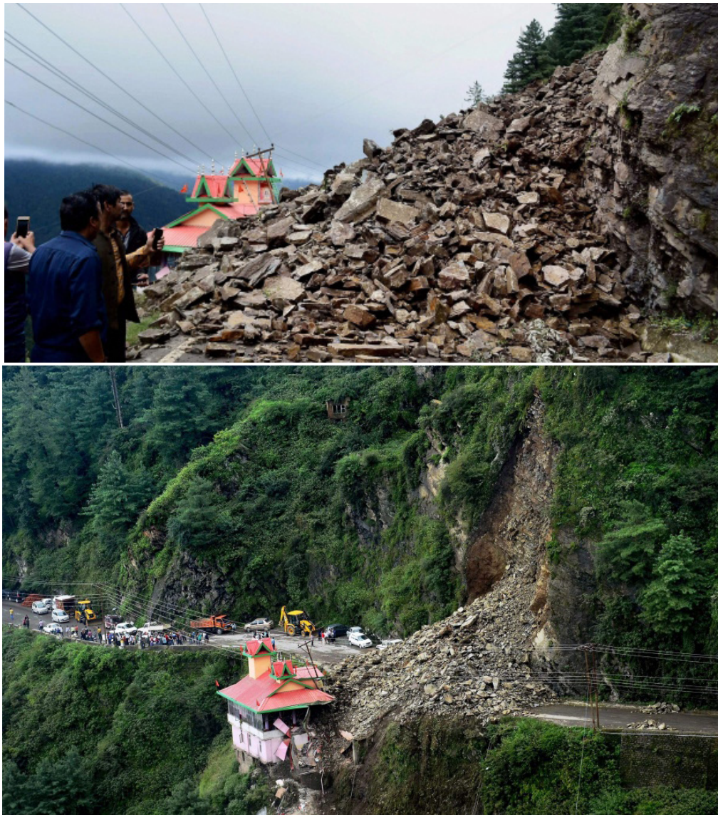
Fig. 6. A view of a major landslide after heavy rainfall in Shimla
