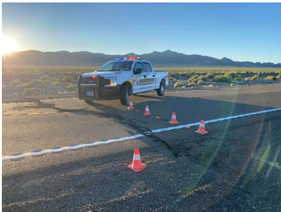
Fig. 2. Esmeralda County Sheriff's Office photo of cracks across Highway 95 ( http://www.nbmj.unr.edu/Geohazards/Earthquakes/MonteCristoRangeEQ.html )
