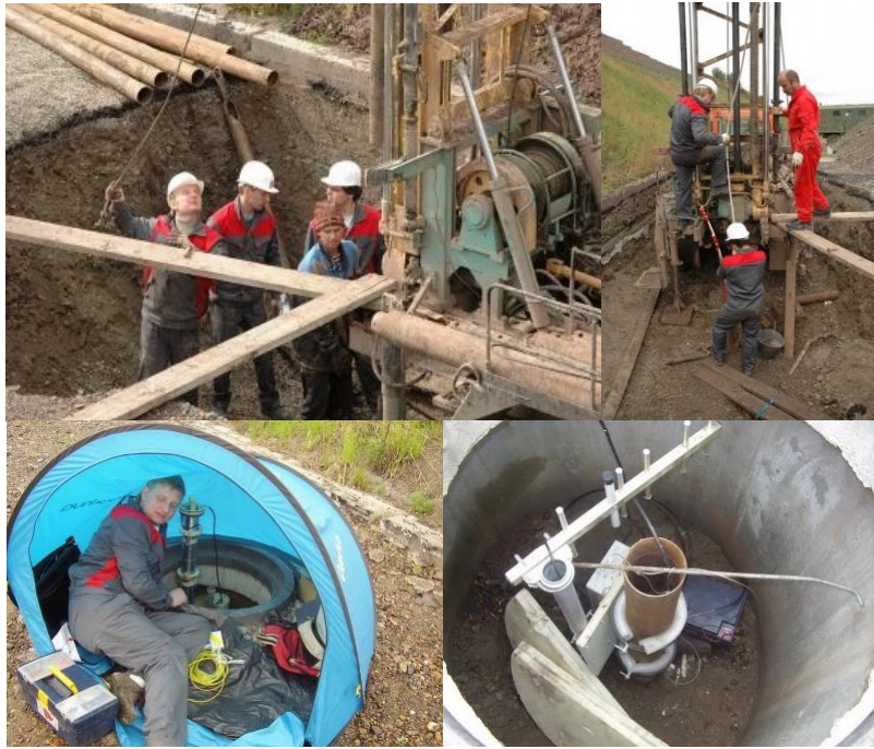
Fig. 2e. Installation and commissioning of geohazards monitoring system (Ginzburg A.A.).
