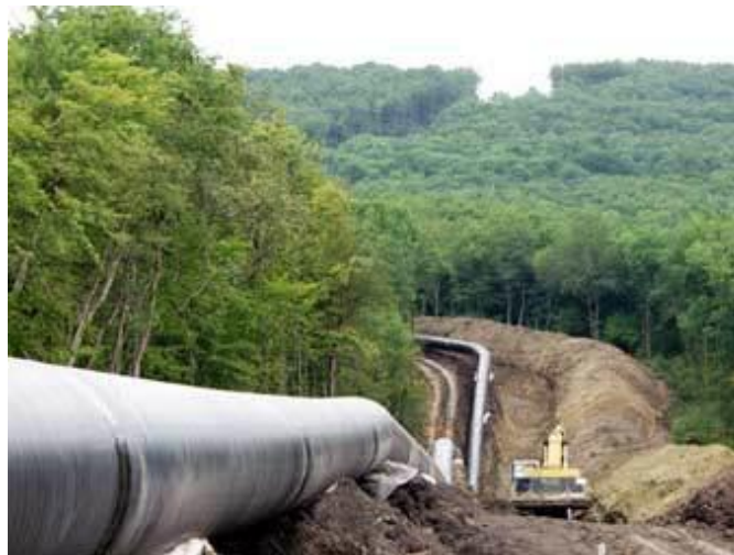
Fig. 4b. "Blue Stream" during construction.
